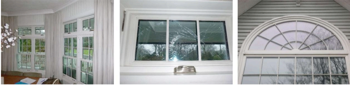
Photos 7, 8, 9: Bottom an top sash windows with hinged vent windows above them, fixed windows half round shaped windows. All with crossbars on both sides.
