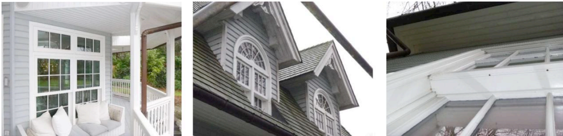
Photos 4, 5, 6: Shielding by canopies, eaves and gutters.
