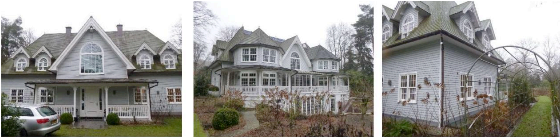
Photos 1, 2, 3: Front side of the villa is facing NNW, backside SSE, right side WSW.
