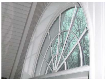
Photo 27: The closeness of the crossbars indicates touching panes and foils.
