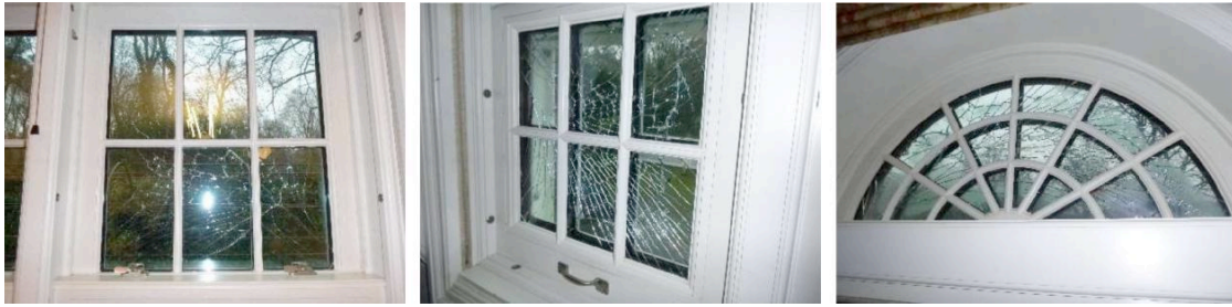
Photos 18, 19, 20: Three imploded units (numbered 4, 5 and 6) with broken inside panes. Situated respectively in a: top sash window ground floor in the office, bottom sash window and half round fixed window both in the same window frame at the first floor bedroom. All units are in the WSW facing (right side) façade.
