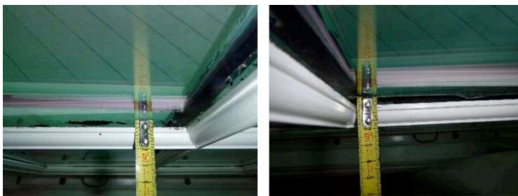
Photos 25, 26: Detached crossbars with 5 mm spacing between crossbar and glass pane.
